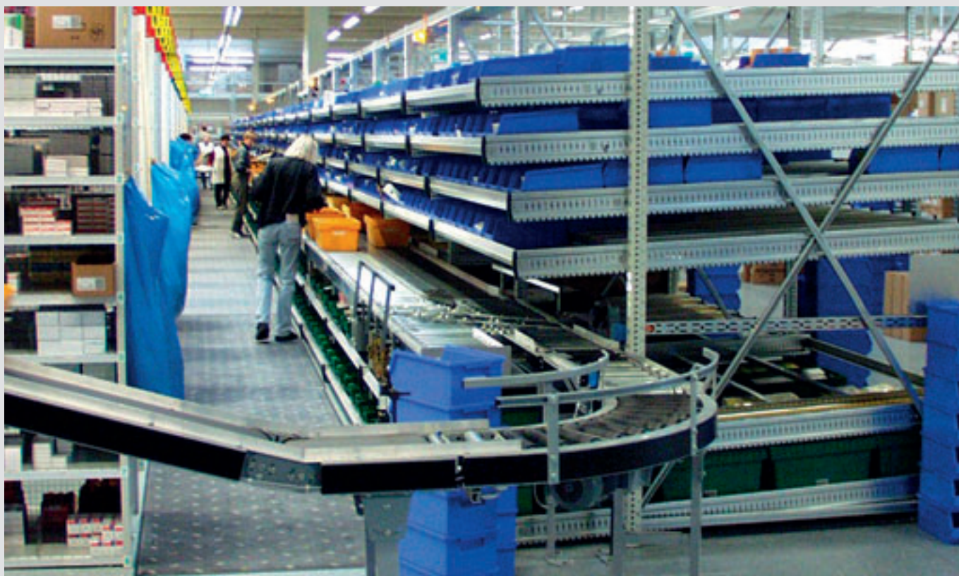
KDR with integrated conveyor system in pharmaceutical wholesale
